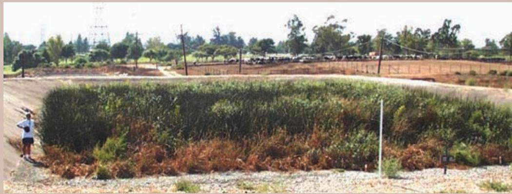
SSF wetland designed to treat dairy washwater in Chino, CA. This front-loading wetland contains 10 percent coarse gravel, 10 percent aquatic grasses to remove solids and 80 percent bulrush to remove nutrients.
